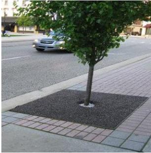
Example of flexible porous pavement
