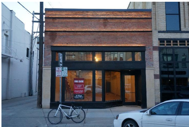
Recently Rehabilitated Façade of 112 N 4 th Street
